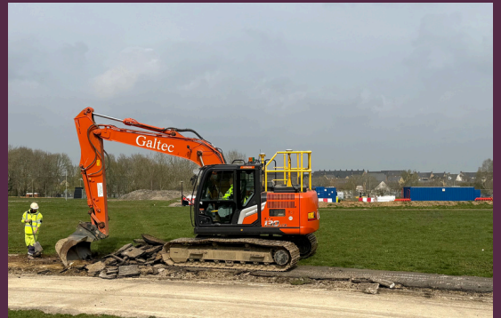
A digger undertaking enabling works at Brize Norton.
